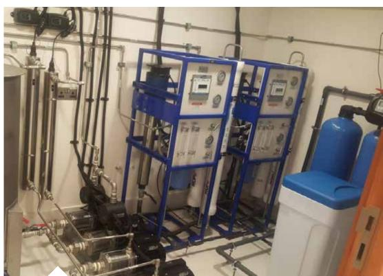
Under our Water Division, SE Dubai installed and commissioned a state-of-art water treatment system at one of the leading hospitals in UAE: Al Zahraa Hospital (Sharjah). The system produces 3000 Gallons/day of ultra-pure water for kidney dialysis purposes - a complete desalination, disinfection & recirculation system that complies with the highest quality standards of water for medical purposes.
